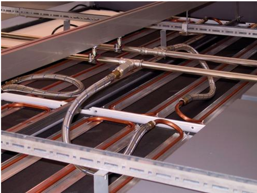
Figure 3. Back View of Drop Ceiling: Piping Configuration with Flexible Hose and Quick-Connect Fittings
