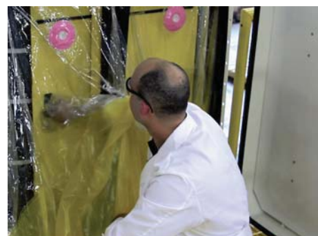
Surrogate tested bag-in/bag-out safe change option available.
