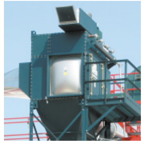
Explosion Vent—NFPA Rupture Panel
