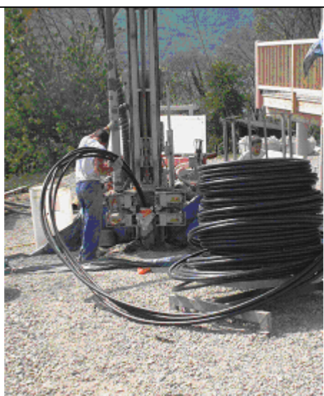
Pipe being inserted into borehole
