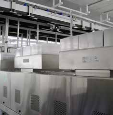
AMC filtration on top of process equipments
