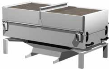
AMC filtration on top of process equipments
