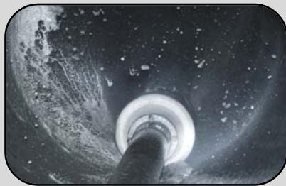
水泥内衬修磨 Grinding in lining
