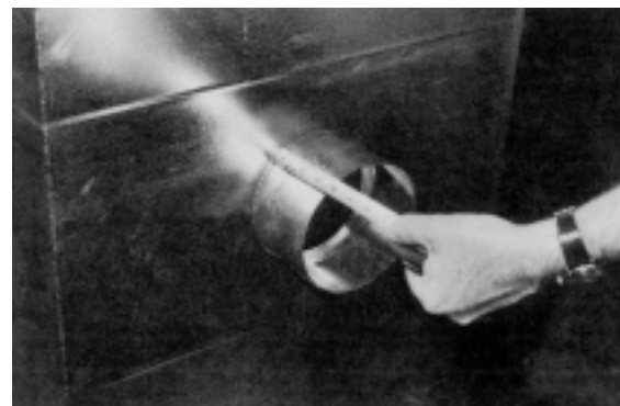
Figure H — Collar in duct min. 2"
