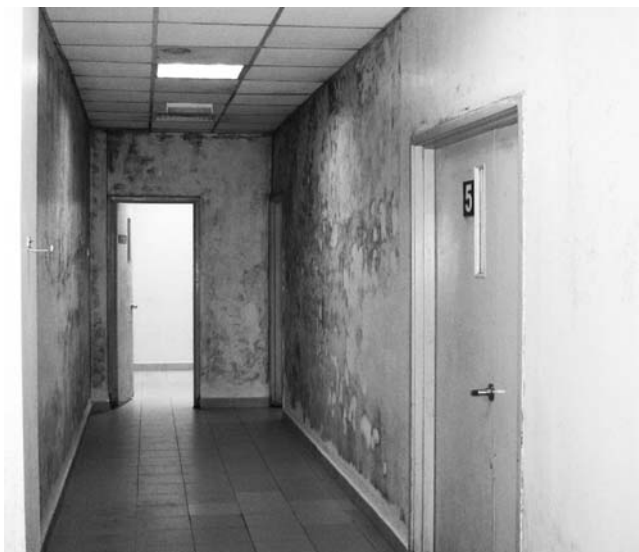
Fig. 4 Mold Resulting from Humid Air Infiltration in Overcooled Health Clinic
