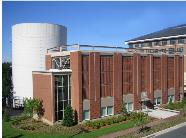
Figure 6.2 The 66,000 ton-h (230,000 kWh) of stratified CHW TES at the University of North Carolina in Chapel Hill, North Carolina, was first in service in 2004. The 85 ft diameter x 116.83 ft high (35.6 m x 25.9 m), 5.0 million gallon (18,800 m 3 ) welded-steel tank, operates at CHW supply temperature of 39°F (4°C) and a return temperature of 60°F (16°C) and was designed for possible future conversion to LTF TES service at a larger DT and increased thermal capacity. In CHW TES service, it reduces peak demand by up to 10,000 tons (35,000 kW) of cooling and approximately 7 MW of electric power (or approximately 40% higher if converted to LTF TES).
