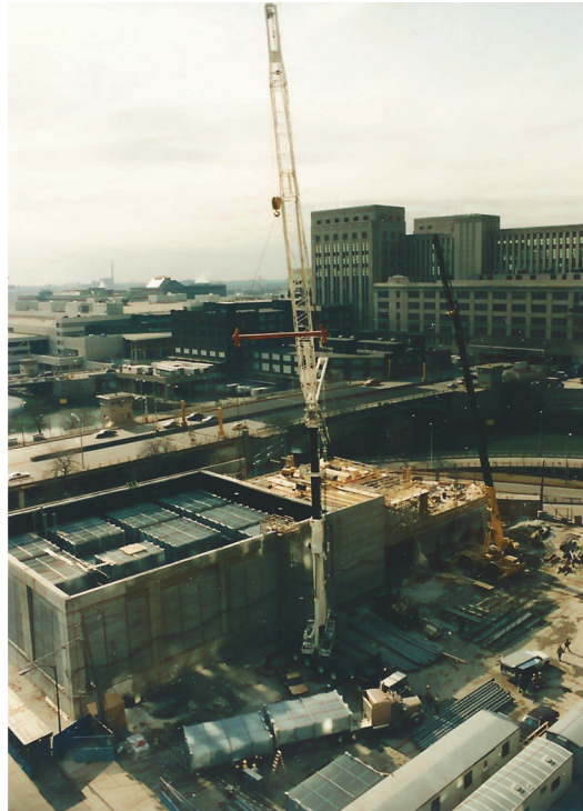
Figure 6.1 The 125,000 ton-h (440,000 kWh) of ice-on-coil TES at Thermal Chicago's District Cooling Plant #2 in Chicago, Illinois, was first in-service in 1996. The 114 ft long × 91 ft wide × 32 ft high (34.7 m × 27.7 m × 9.8 m), 2.5 million gallon (9,400 m 3 ) concrete tank, holding 144 ice-on-coil modules, operates at a nominal water-glycol charging (ice building) temperature of 20.5°F (−6.4°C), and a water discharging (ice melting) temperature of 34°F (1.1°C). It can reduce peak demand by up to 14,600 tons (51,000 kW) of cooling and approximately 10 MW of electric power.
