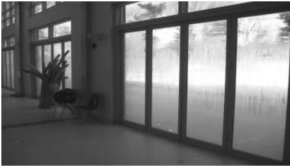
Figure 5. Condensation on Windows: Glass Surface Is below Space Dew Point
