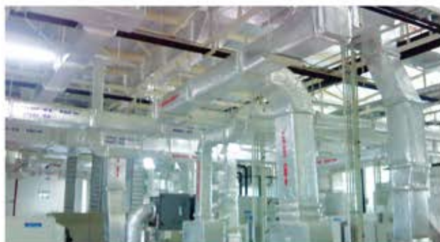
Neat appearance when used as external insulation for air ducts in pharmaceutical laboratory facility.
