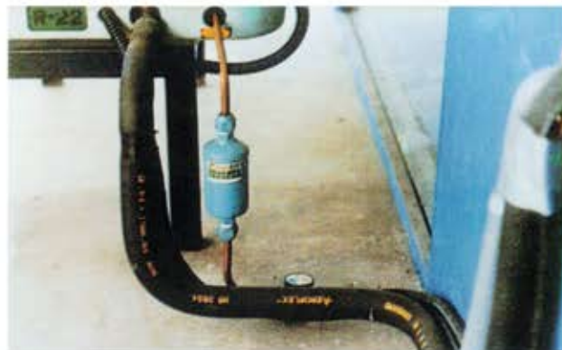
Flexibility and outstanding durability, Aeroflex is the most suitable insulation for split type air-conditioners.
