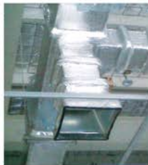
Aeroflex can work efficiently as a sound dampening material when used as internal and external insulation for medium and high velocity air duct system.
