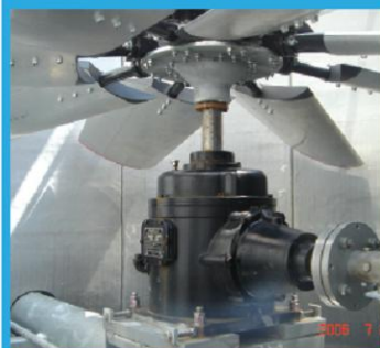
Gear Reducer Drive System
