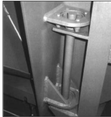
Heavy duty ball bearings provide door support.
