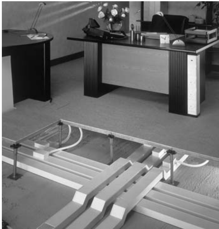
Fig. 4.1 Installed underfloor trunking. Note the segregated circuits.
