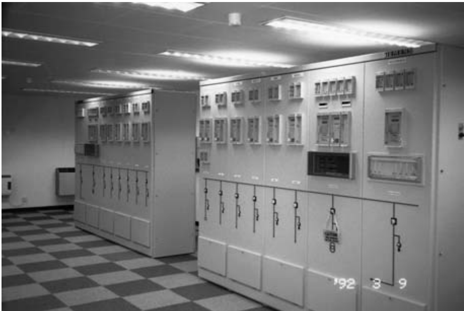
Fig. 2.2 Digital control panel, Jersey ( Siemens plc ).
