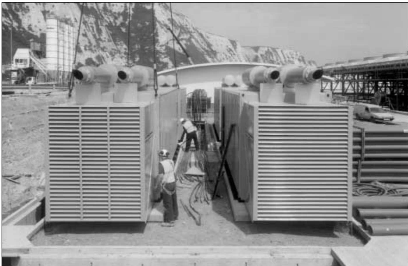
Four 1250kVA automatic starting, auto sync sets in specially adapted containers reduce noise levels down to 75dB(A)@1m Photo: Courtesy of EuroTunnel - Transmanche link
