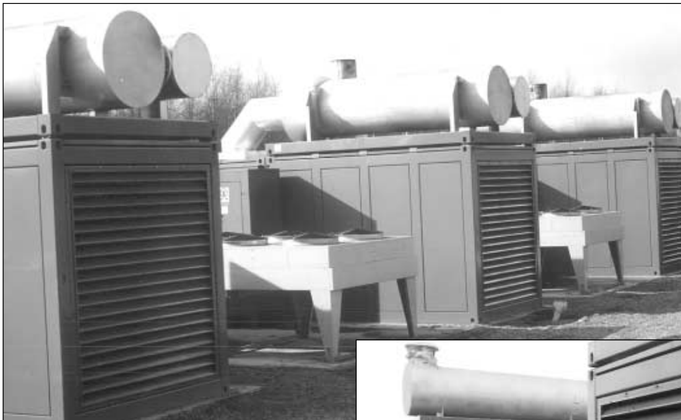
Three containerised, 2.2 MW HV sets used for peak lopping duties with horizontal external cooling radiators. Whole installation silenced down to 75dB(A) at 1m and inaudible at around 50ft.
