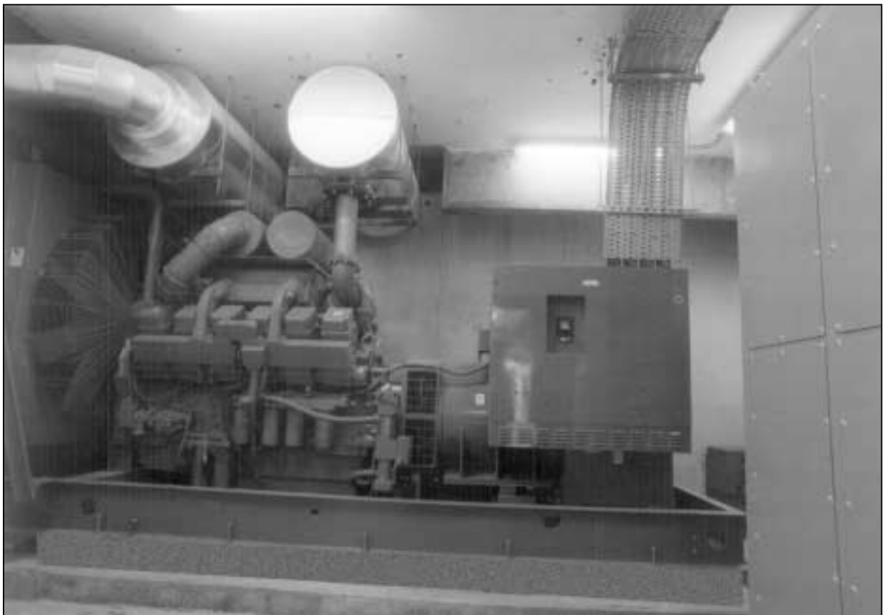
Top cable entry. Control panels provide choice of top or bottom entry. LH or RH mounted.
