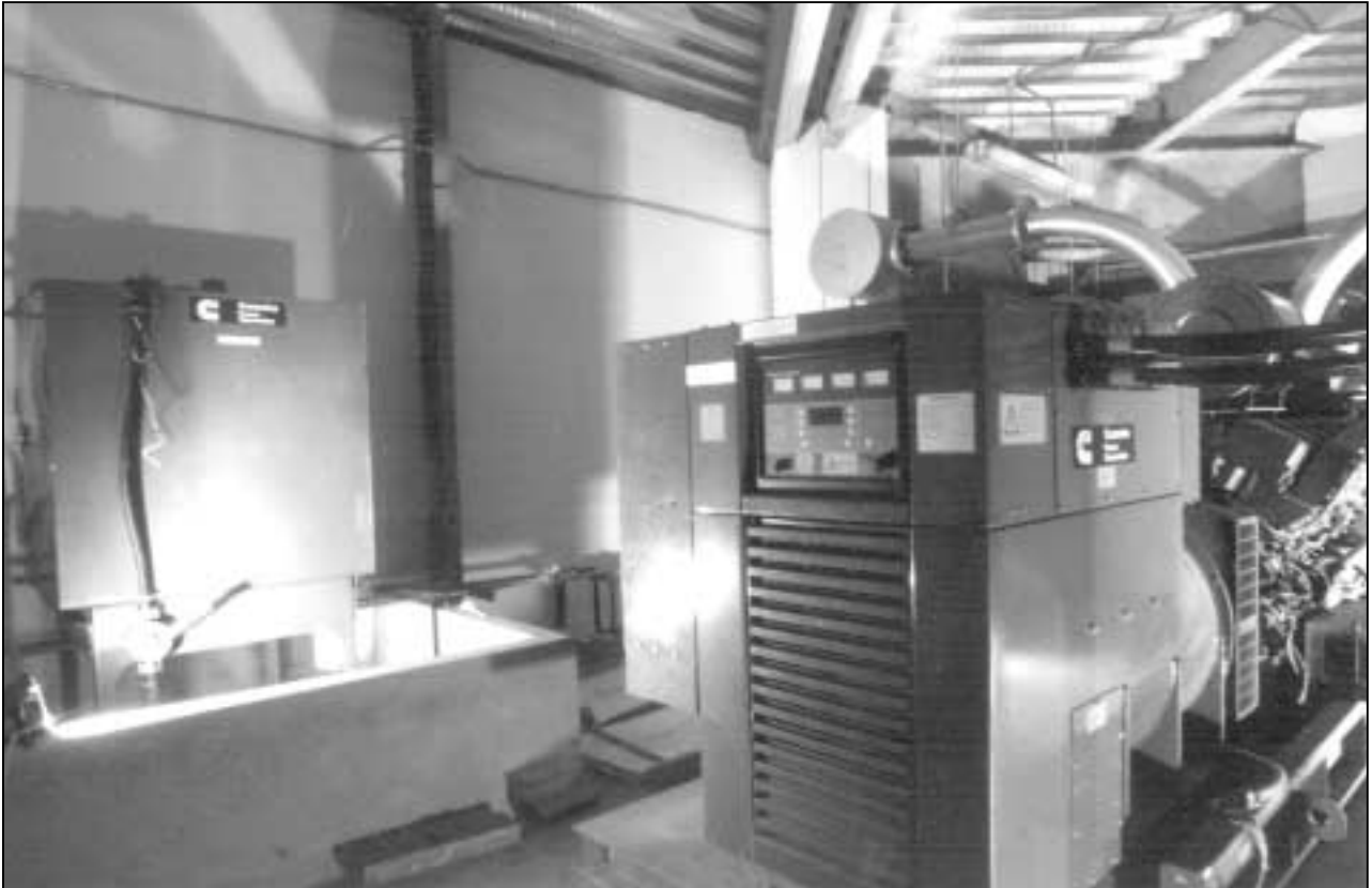
Example of a free standing 900 Litre fuel tank installed within a bund wall.
