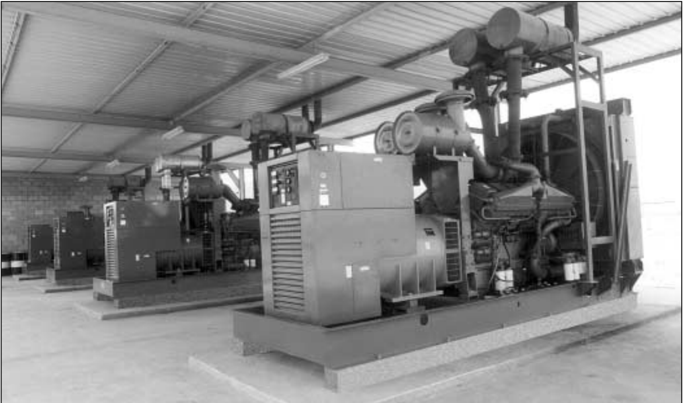
4 x 800 kVA Gen Sets in a ground level room installation with simple but effective exhaust run.
