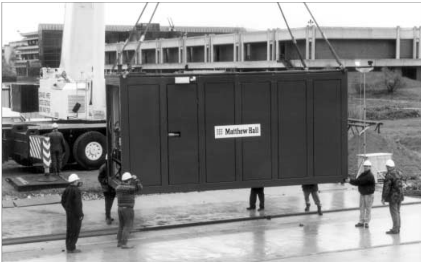
6m (20ft) silenced module forms part of an 18m (60ft) installation containing a 2000kVA standby generator
