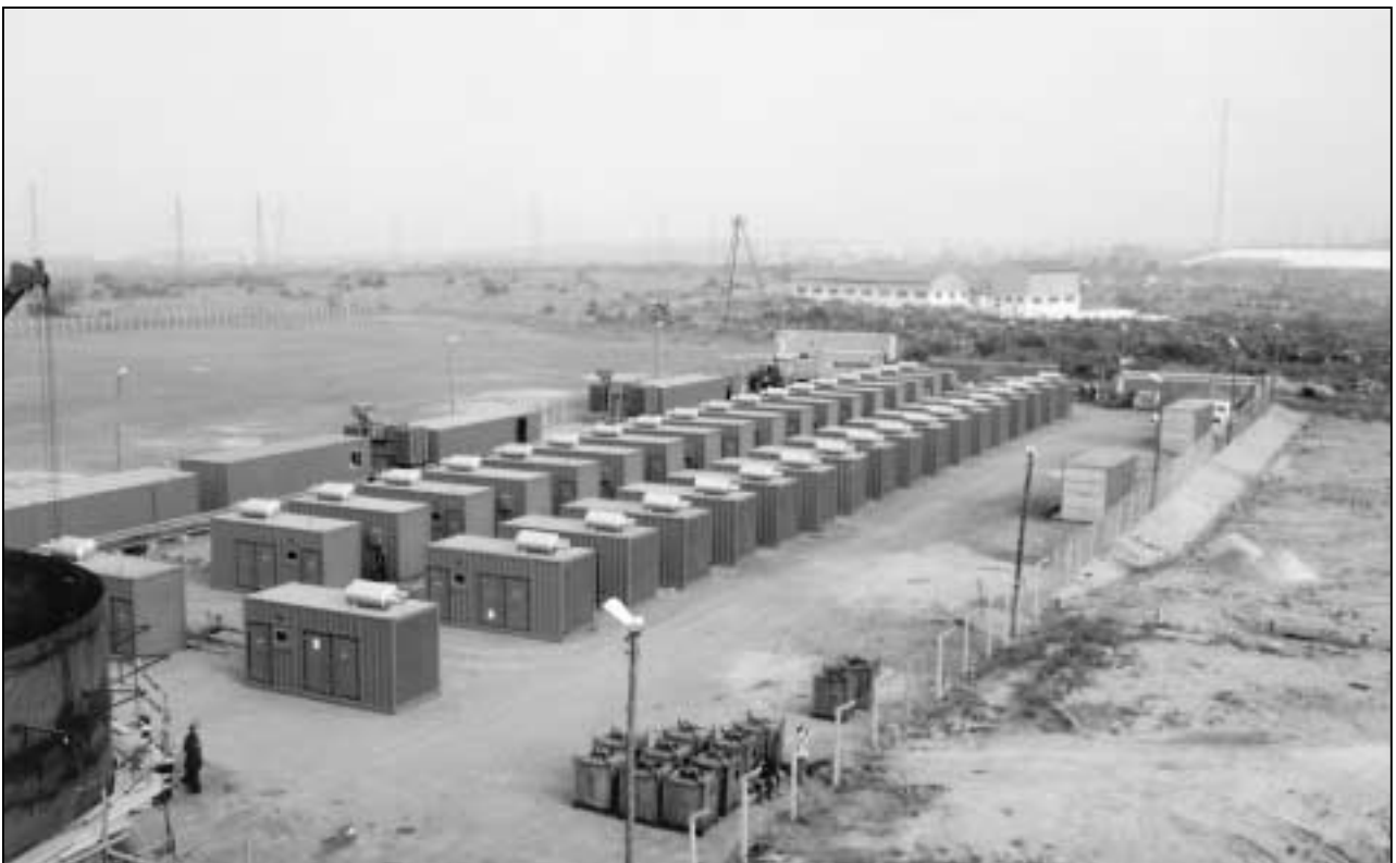
Thirty-nine 1125 kVA sets with KTA50 engines produce a combined 30MW of site power using PowerCommand Control (PCC) and Digital Master Control Systems when all operating in parallel.
