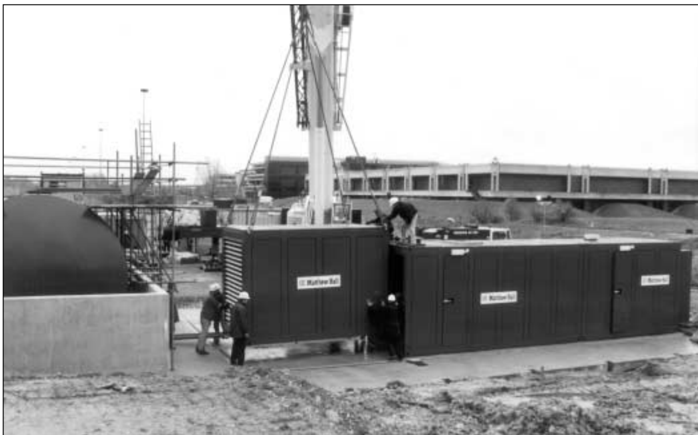
Modular construction cuts time factor down significantly on site.
