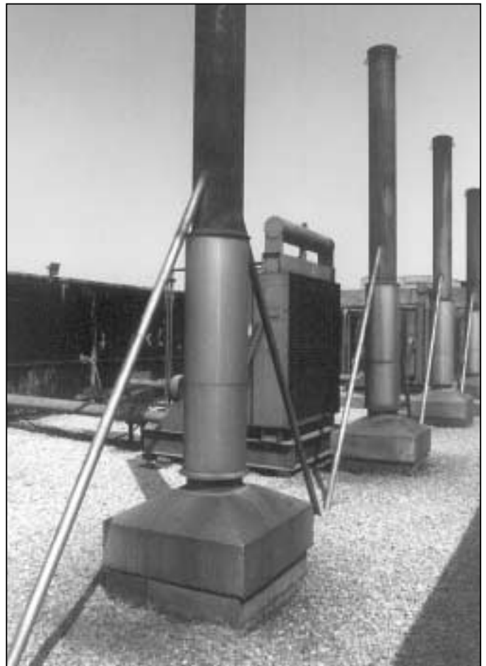
Roof mounted remote radiators for four 1000 kVA sets and extended exhaust tail pipes where space and air flow is restricted.
