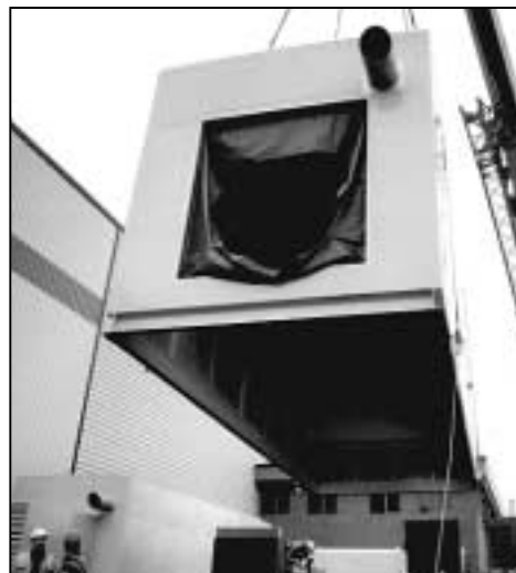
Drop over super silenced enclosure for 2 x 1000 kVA standby generators.
