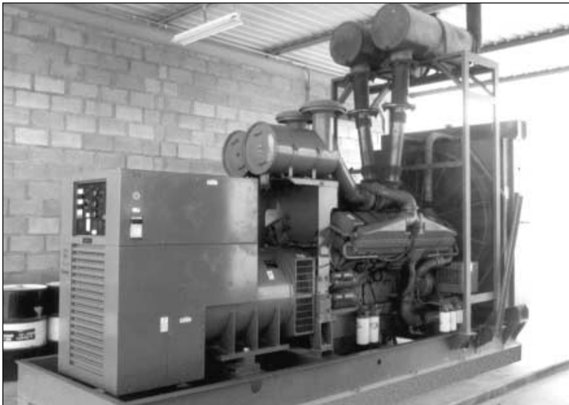
Model CP625-5 (640kVA) in a typical hot climate installation.
