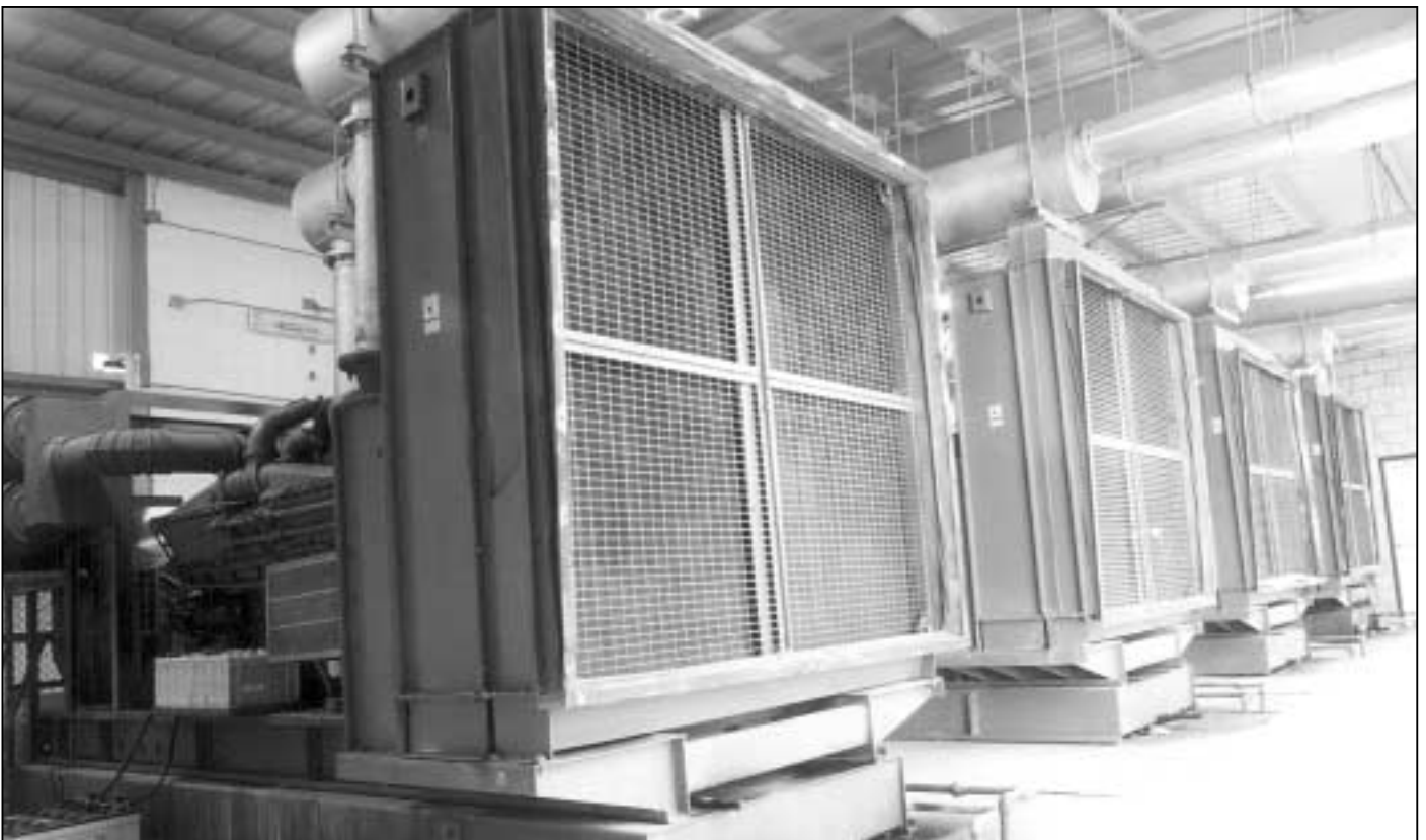
Four 1500 kVA sets with KTA50 engines running on base load operation in Saudi Arabia.
