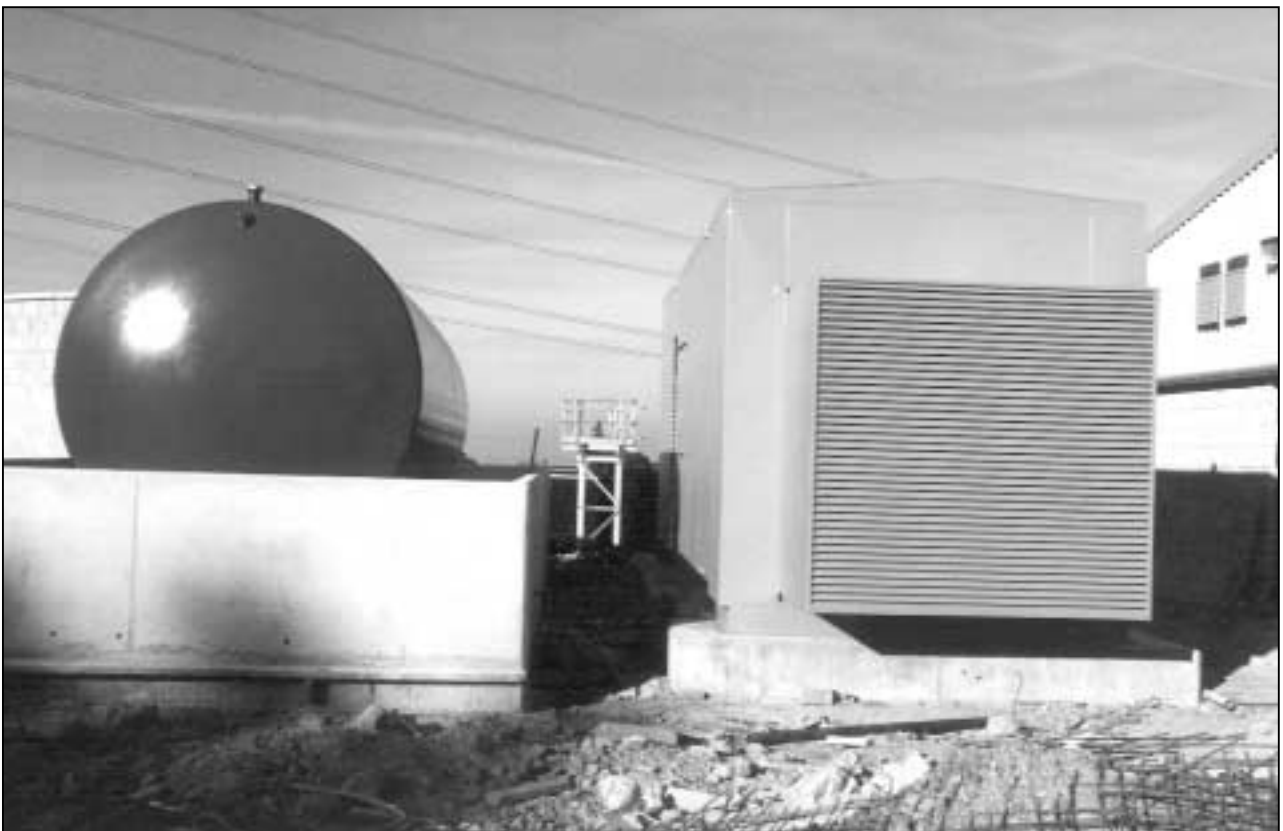
14000 Litre (3000 gallon) bulk fuel tank with a bund wall. Feeding a 500 kVA super silenced set with sufficient fuel for 6 days full load operation.
