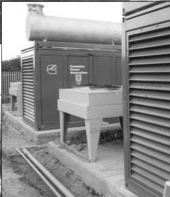
6.6 MW installation. Fuel piping and auxiliary cabling runs.
