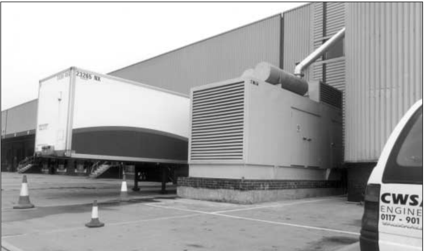
1000kVA Super Silenced (75dBA @ 1m) automatic standby set for major hypermarket chain warehouse
