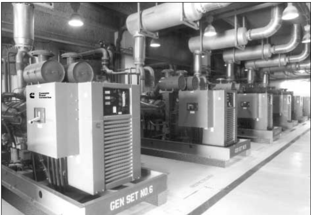
Seven 900 kVA sets working in parallel for a major soft drinks bottling factory in the Middle East.
