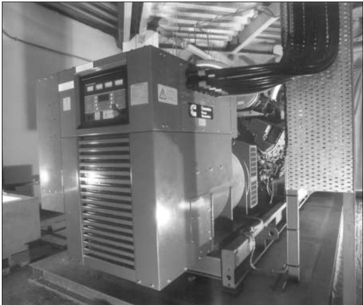
Flexible cable entry into control module and cable tray arrangement for side entry.
