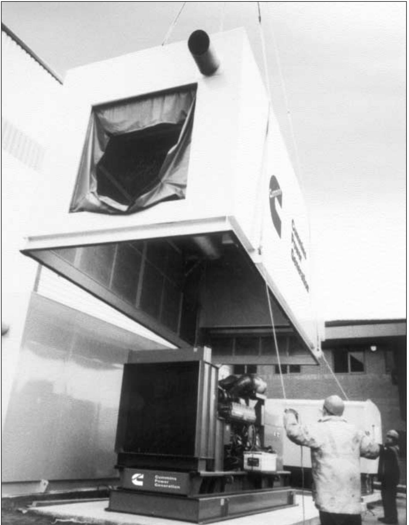
Fig. F1 A typical drop over Acoustic Enclosure for a 1000 kVA generator.
