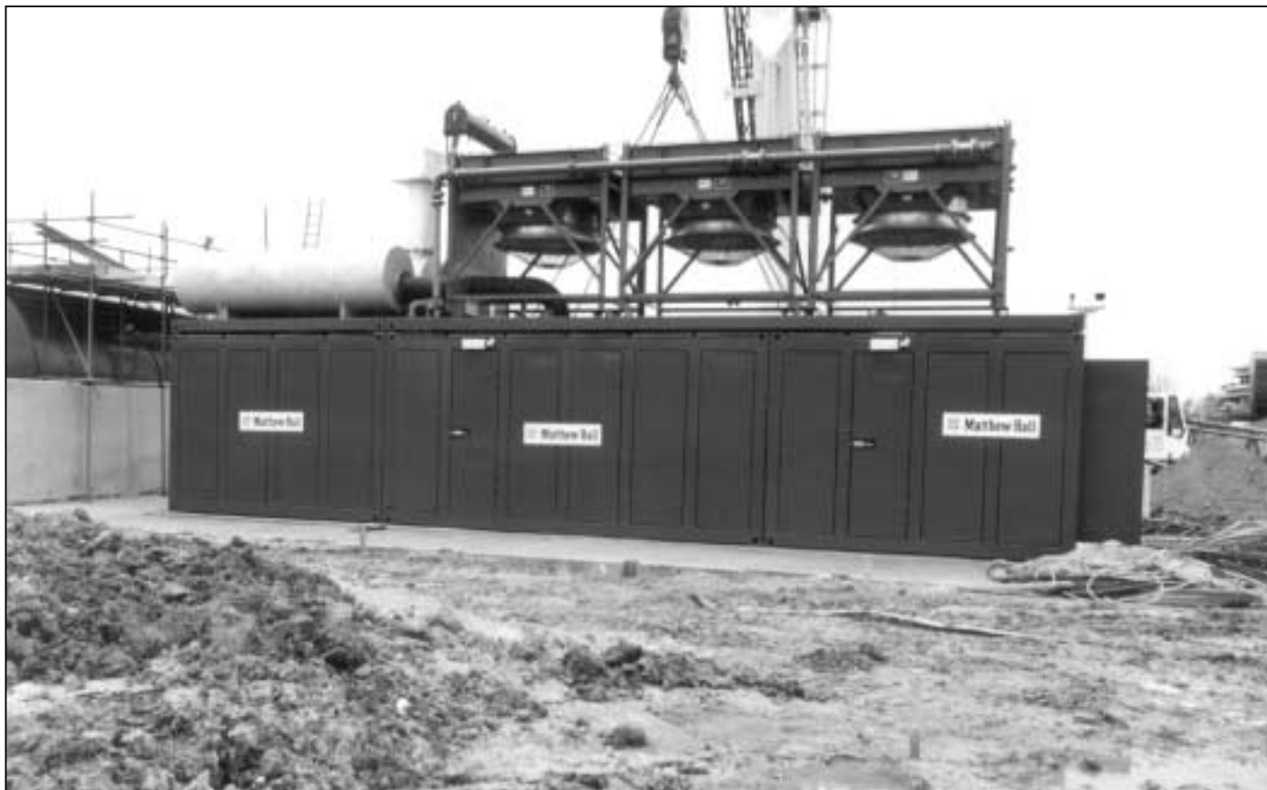
Completed installation with roof mounted radiators and exhaust system.
