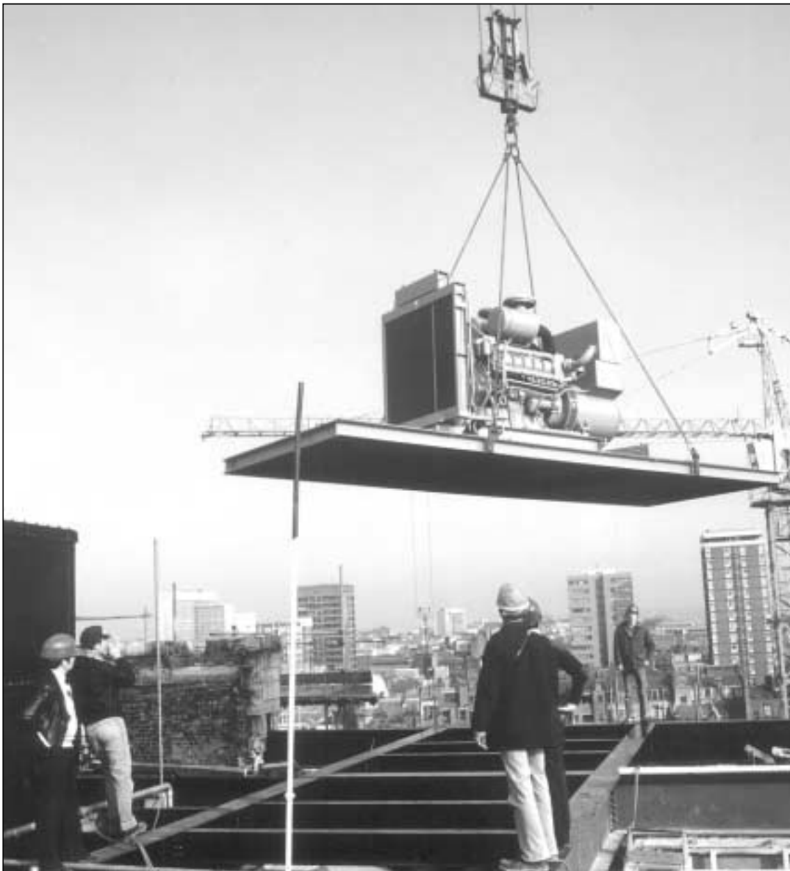
Where possible a packaged set, 300 kVA as shown in picture, on a base frame provides a faster installation. Silenced enclosure drops over unit. Note prepared steel structure support base.
