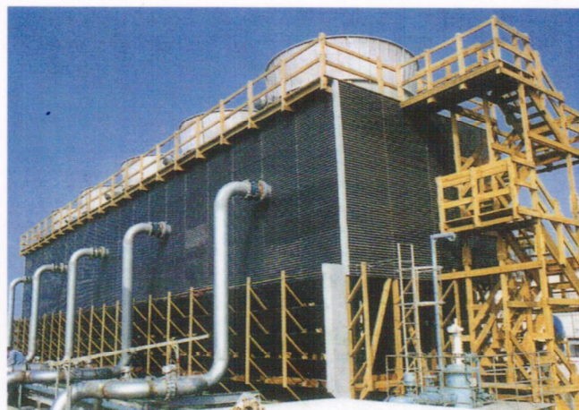
Wood Structure Counterflow
