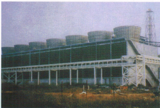
Concrete Structure Crossflow
