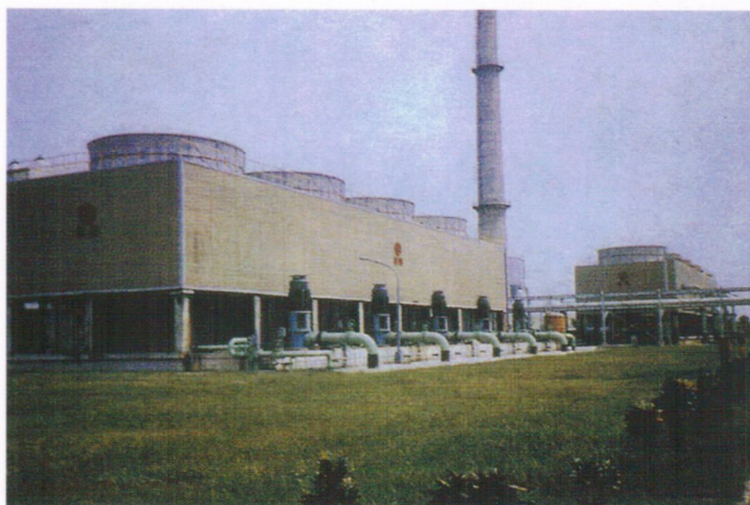
Concrete Structure Counterflow
