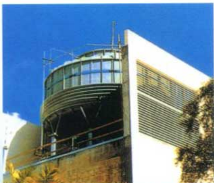
KST-1500x4 KST-1250x2 KST-1000x2 ABOVE 8 UNITS KST COOLING TOWERS ARE OPERATING IN MIAMI BEACH CONVENTION CENTER. PICTURE SHOWS ONLY ONE OF THEM
