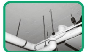
1 FLUSH MOUNTED FIXING WITH INTERNAL THREAD
