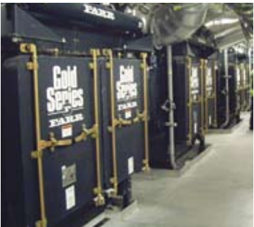
Multiple GS Dust Collectors on Tablet Coaters
