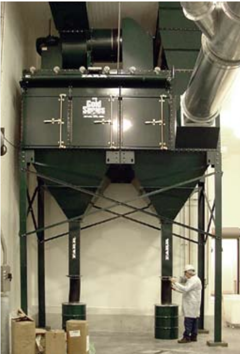
GS24 Connected to SS Hoods Below on Spice Dust Collection
