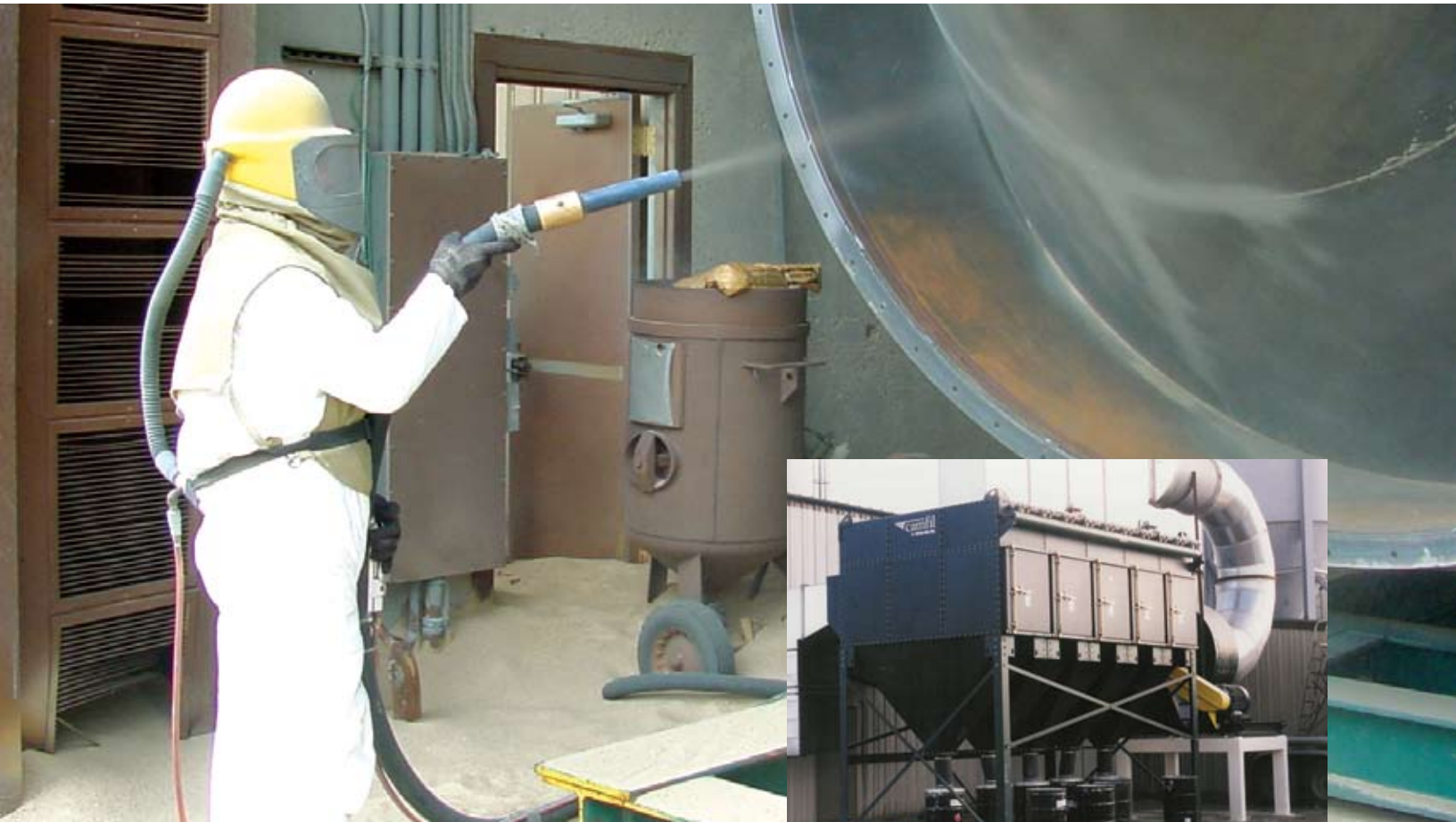
GS60 on Windmill Tower Grit Blasting
