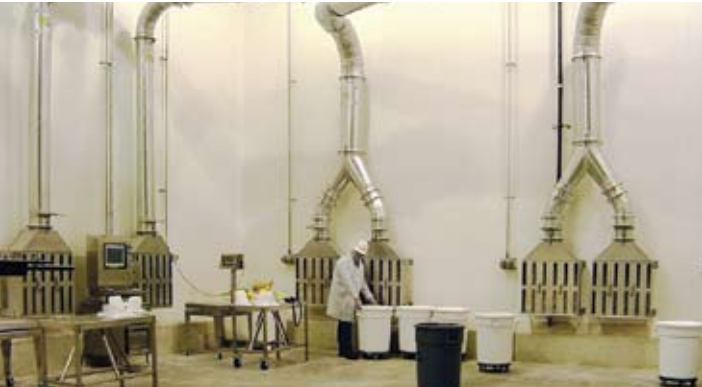
SS Side Draft Hoods for Spice Weighing
