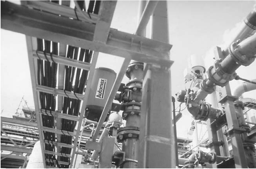
Figure 1.3 Quarter-turn plug valve with rack and pinion actuation system in chemical service. (Courtesy of Automax, Inc. and The Duron Company, Valve Division)
